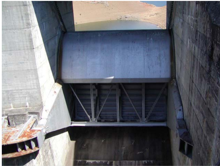
Photo 1. Radial Gate designed to accommodate overflow, Fontana Dam, NC.
