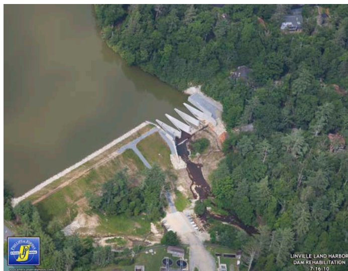
Photo 9. Linville Land Harbor Dam: labyrinth replacement spillway
