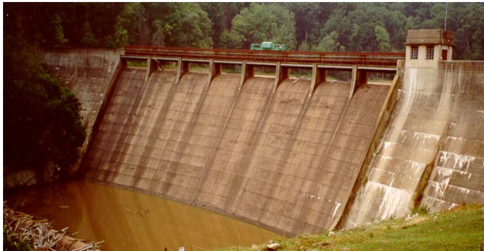
Photo 5. Sugar Hollow Dam: original gated spillway and hoisting system
