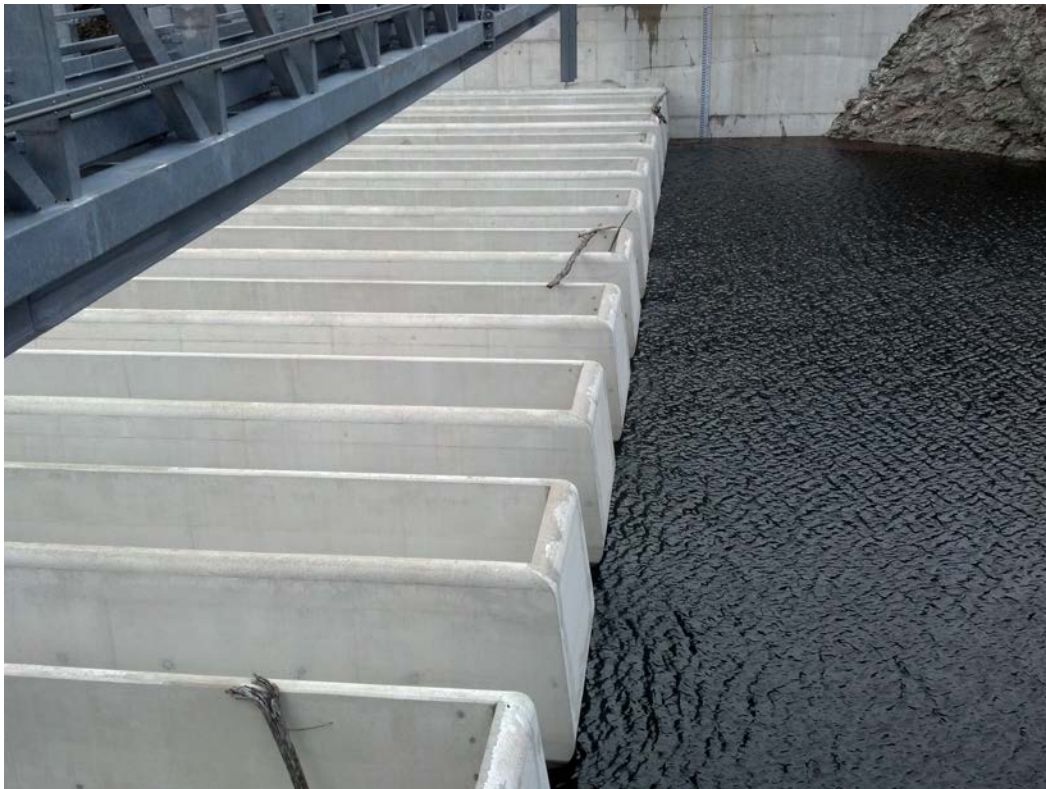
Photo 4. Piano key weir at Malarce Dam
