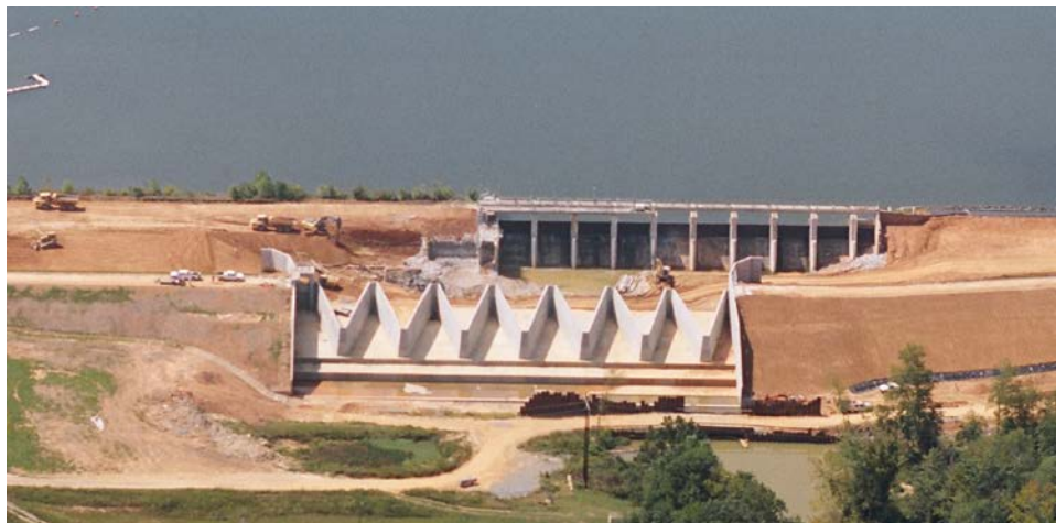
Photo 7. Lake Townsend Dam: Labyrinth spillway constructed downstream of original gated spillway
