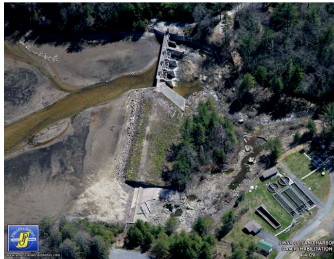
Photo 8. Linville Land Harbor Dam: original spillways
